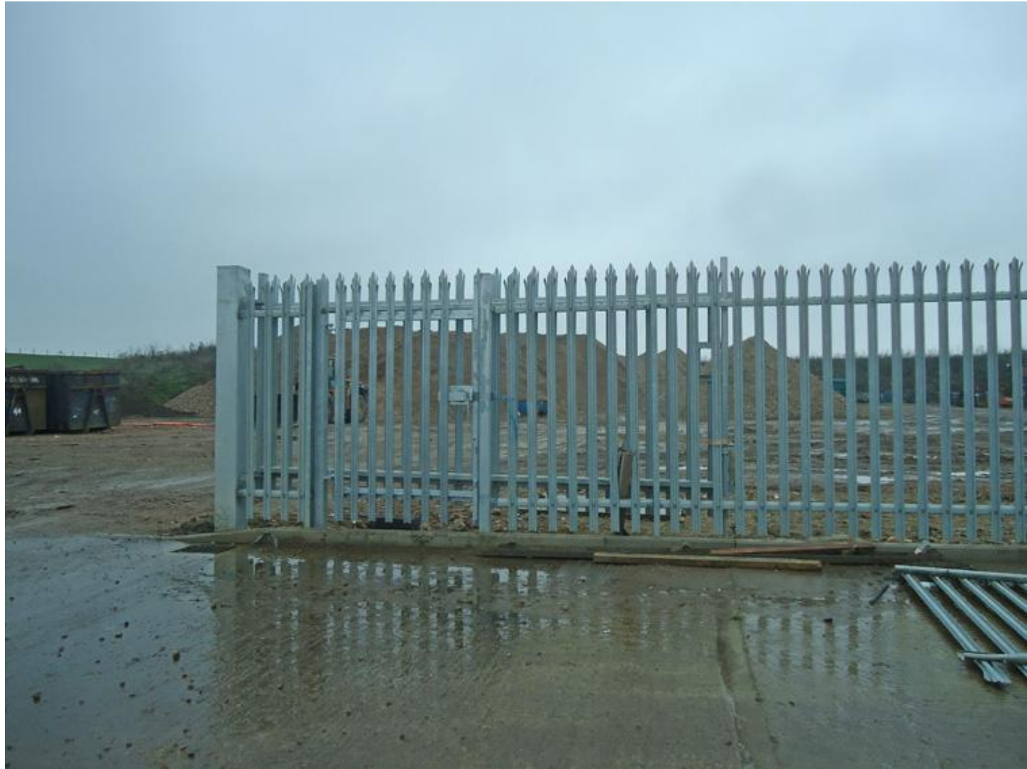
Figure 2 : Unmade surface vs existing concrete facing west (southern extract)
